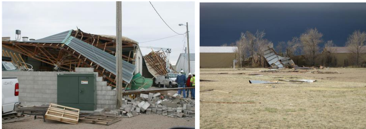
Figure 4.13. Severe Wind Damage in Phillips County (2008) and Yuma County (2009)
